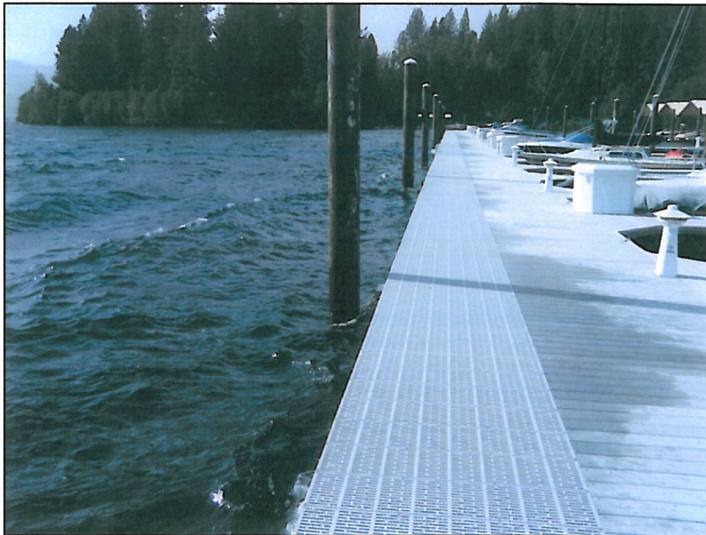
Carlin Bay Property Owners Association Marina HDB Breakwater During Wind Storm
